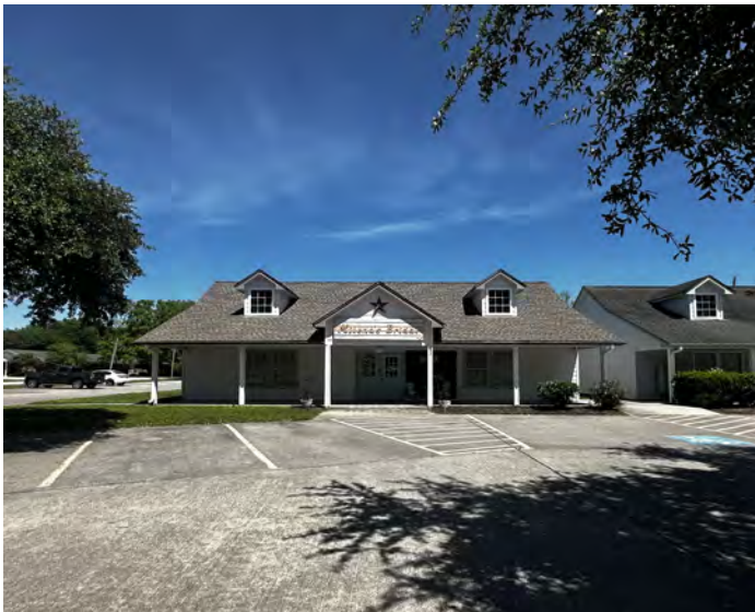
Building B Exterior
