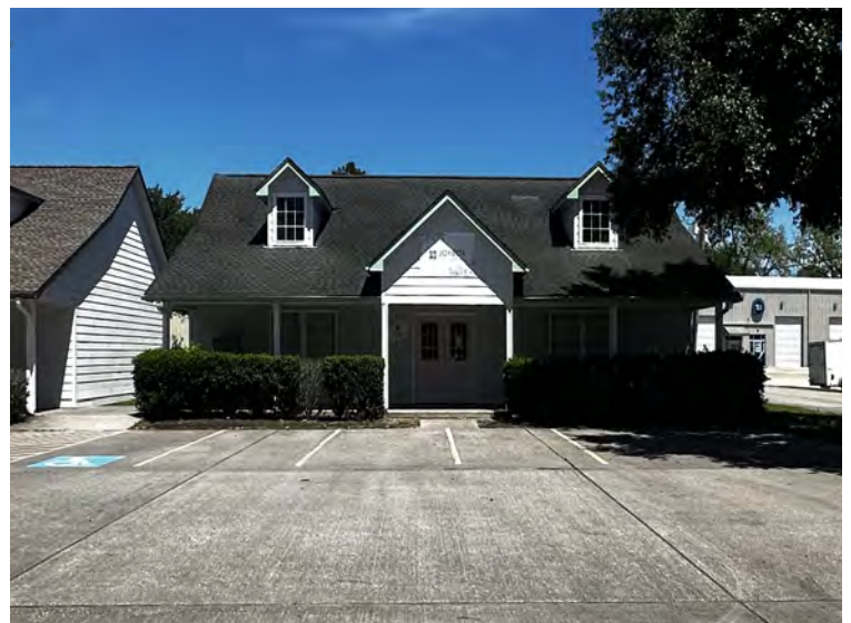
Building A Exterior
